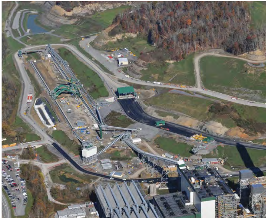
The coal handling operations consist of a truck dump and a stockpile area with linear luffing stackers and rake reclaimers.
