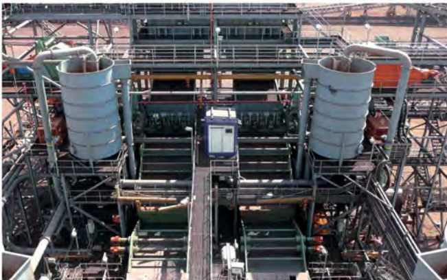
Assmang KEP / South Africa, iron ore beneficiation by using BATAAC jigs
