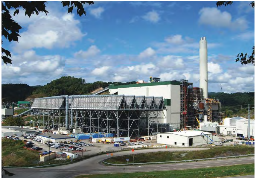
One of the newest power plants in America, the Virginia City Hybrid Energy Center will co-fire bio-mass with coal.
