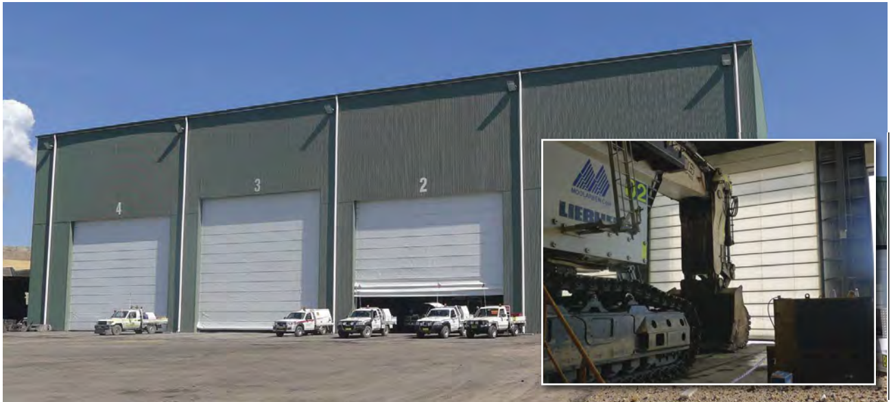
The shop doors seal the opening and they are made from translucent fabric giving the facility more light.
