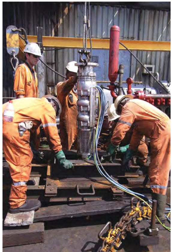
Installing one of Oddesse's innovative dewatering pumps.
