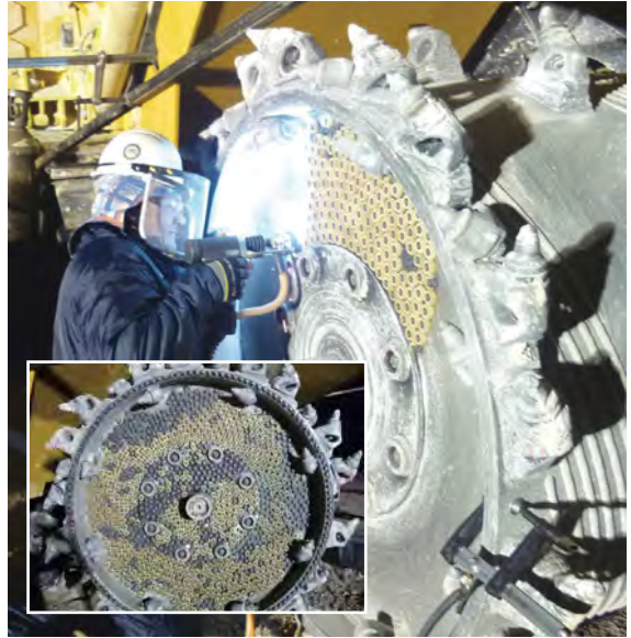
Welding Betek TungStuds as wear protection for a cutting drum.
